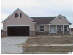
The Wilshire under construction
